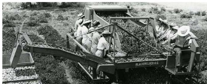
1962- First commercial harvester Required 12 people to operate
